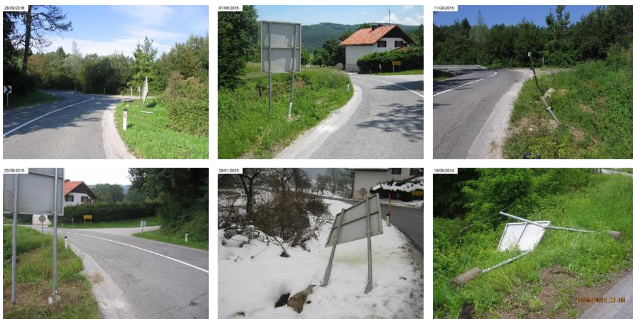
“Figure 5 – Frequented damage of traffic sign”
