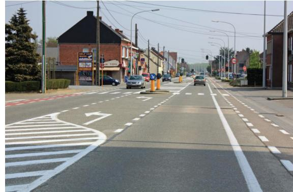
*Picture 8: Linear settlement with traffic calming and improved road side*
