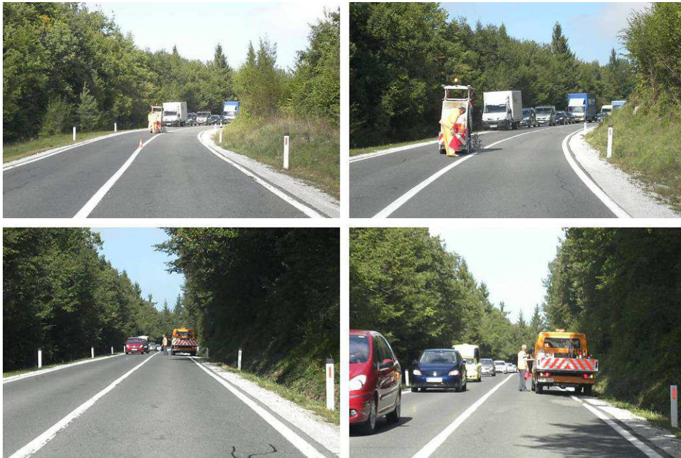
Figure 21 - The effect of sun glare on visibility (Sun glare can reduce the visibility and conspicuousness of signage, workers etc.)
