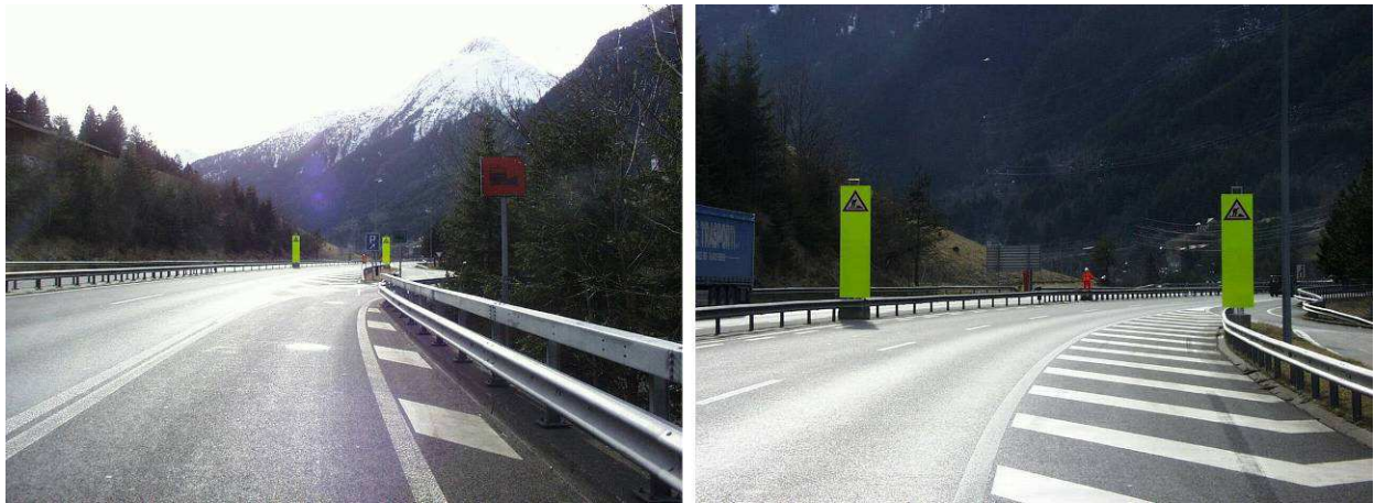
Figure 9 - Conspicuous traffic signs [3] (Alerting driver of road works ahead)
