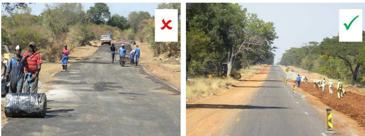
Figure 2 - Pictures shows unclear vs. clear work zone and workers (On right picture driver knows where to drive and recognizes the workers)
