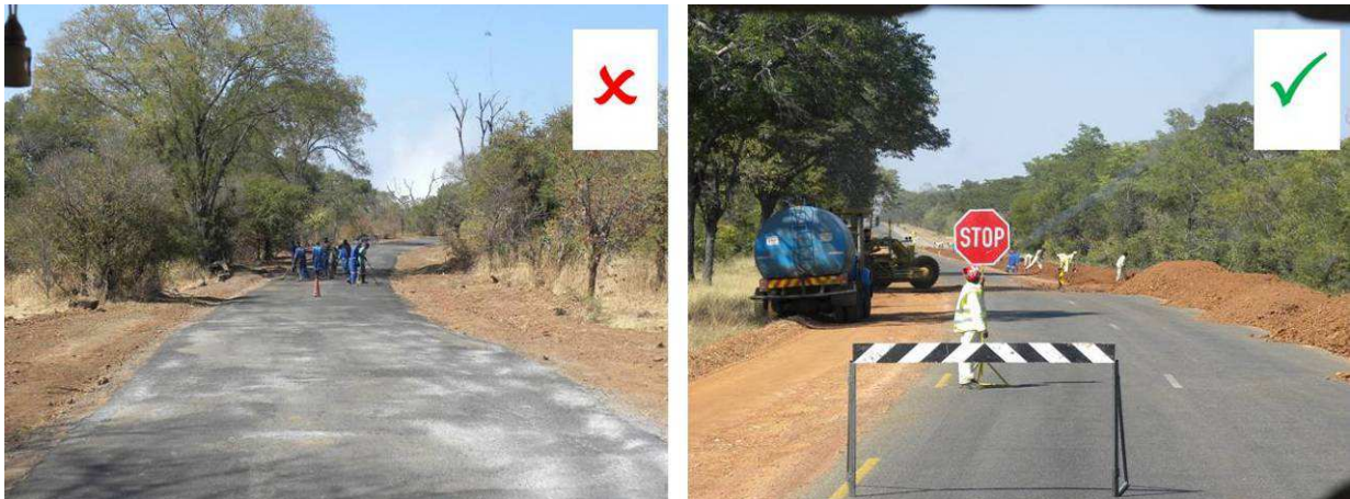
Figure 1 - Pictures shows inconspicuous vs. conspicuous work zones and road workers (TTM on right picture enables driver to see and re-act on time)
