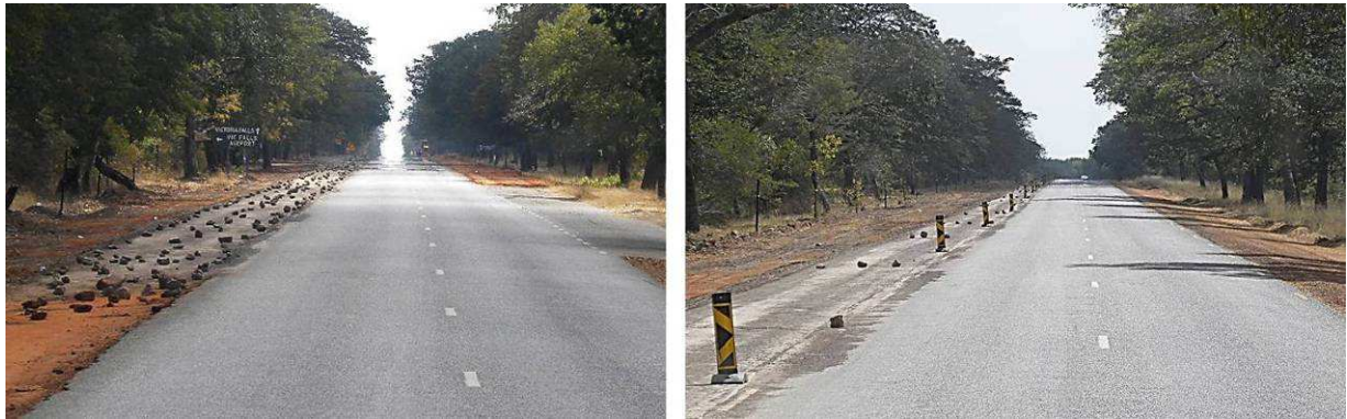
Figure 23 - Preventing driving by using available resources (Placed stones prevent driving on newly laid asphalt and ensure workers safety)
