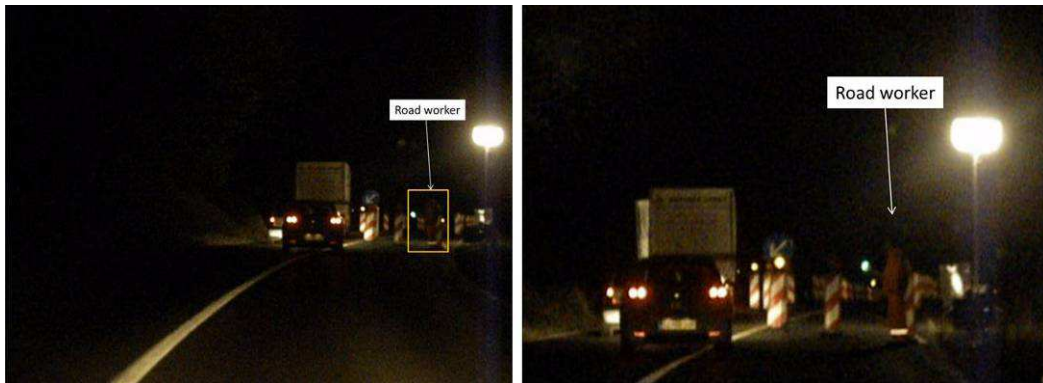
Figure 27 - Illumination and visibility of road worker during the night (Improper illumination dazzles drivers and does not assure the visibility of a road worker)
