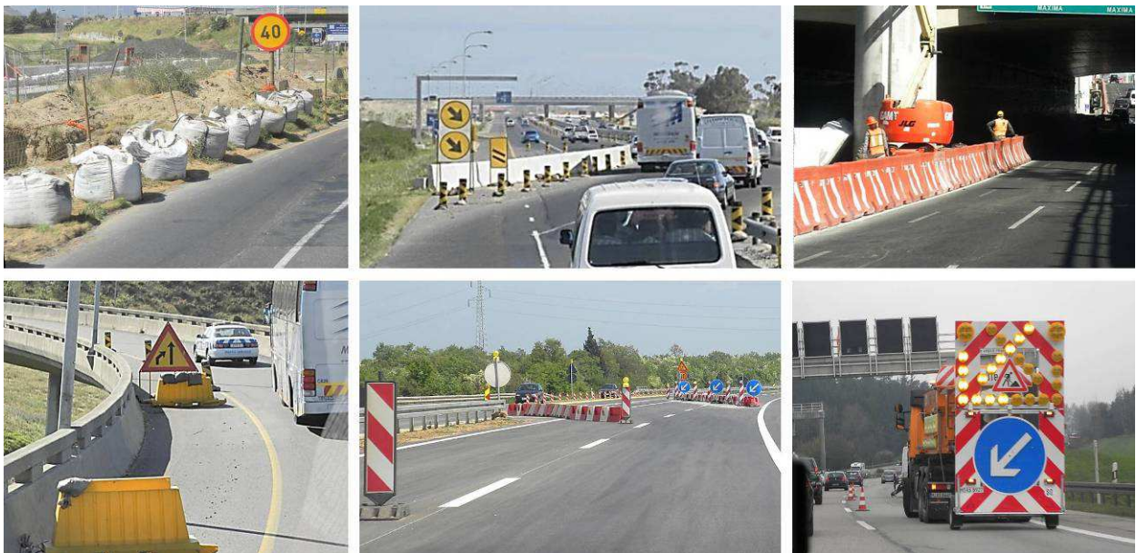
Figure 16 - Physical protection for the road workers and traffic guidance (Variety of ways to protect the workers by separating and calming down traffic)
