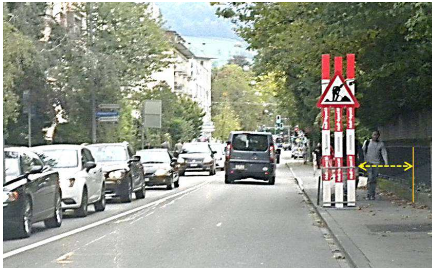
Figure 25 - Conspicuousness of temporary traffic signs and ensuring width for pedestrians
