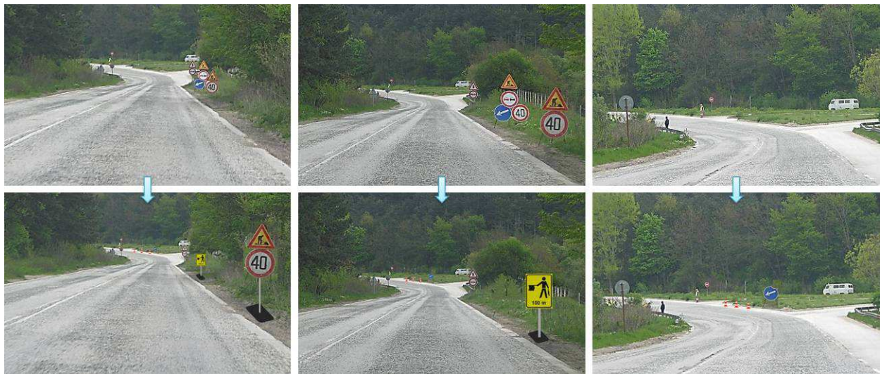
Figure 19 - Clear information of road works ahead (Cluster of traffic signs vs. clear and credible information)
