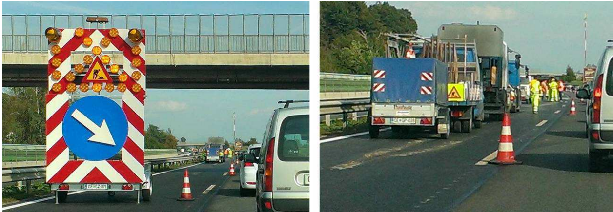
Figure 15 - Buffer zone and side distance (Protection of workers with a traffic trailer with buffer zone and side distance provided by traffic cones)
