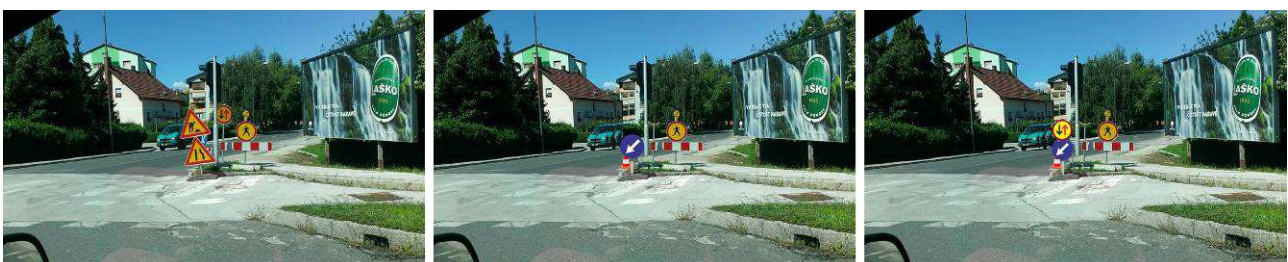
Figure 26 - Clear and comprehensive temporary traffic signage (Driving rules state that in this kind of situation vehicle with obstacle on its way has to give priority to oncoming traffic so additional sign “priority of oncoming traffic” is not required)
