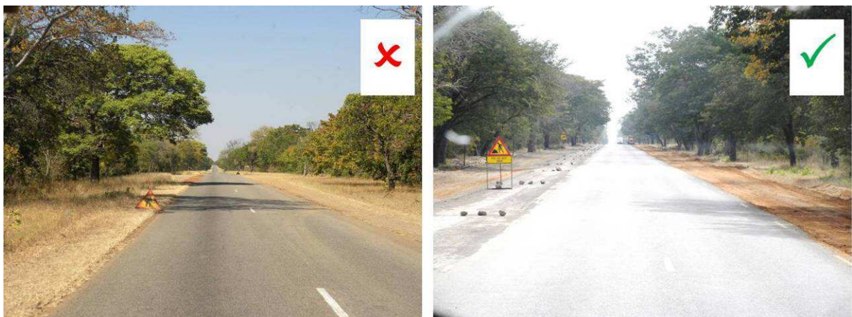
Figure 4 - Pictures shows difference in credibility (On left picture there are no road works after the traffic sign, while on right picture after the sign there are actual road works ahead)
