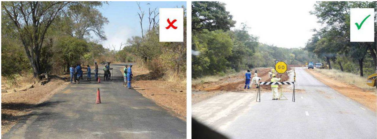
Figure 3 - Pictures shows the difference of consistency (Different principles of traffic arrangements for manual traffic management just a few kilometres apart)
