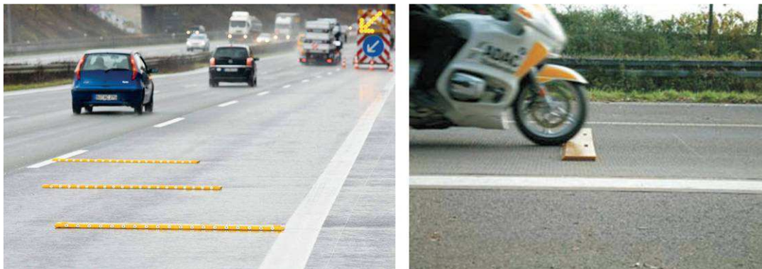
Figure 24 - Warning ramp / tactile road equipment [5] (Traffic equipment for warning and slowing down drivers)
