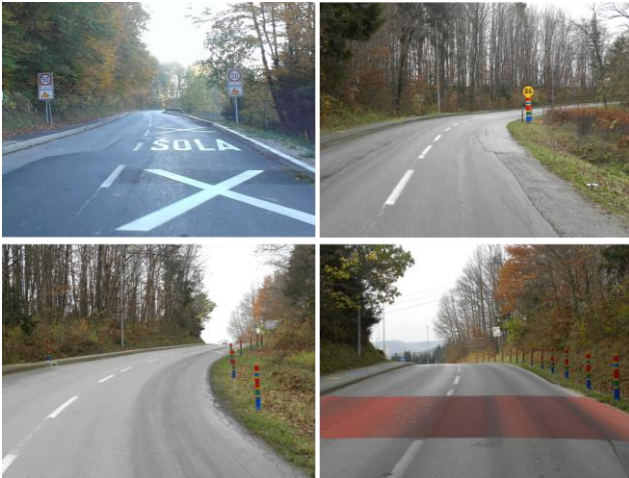
Figure 9: Improved road design in the vicinity of School and Kindergarten (direction "B")
